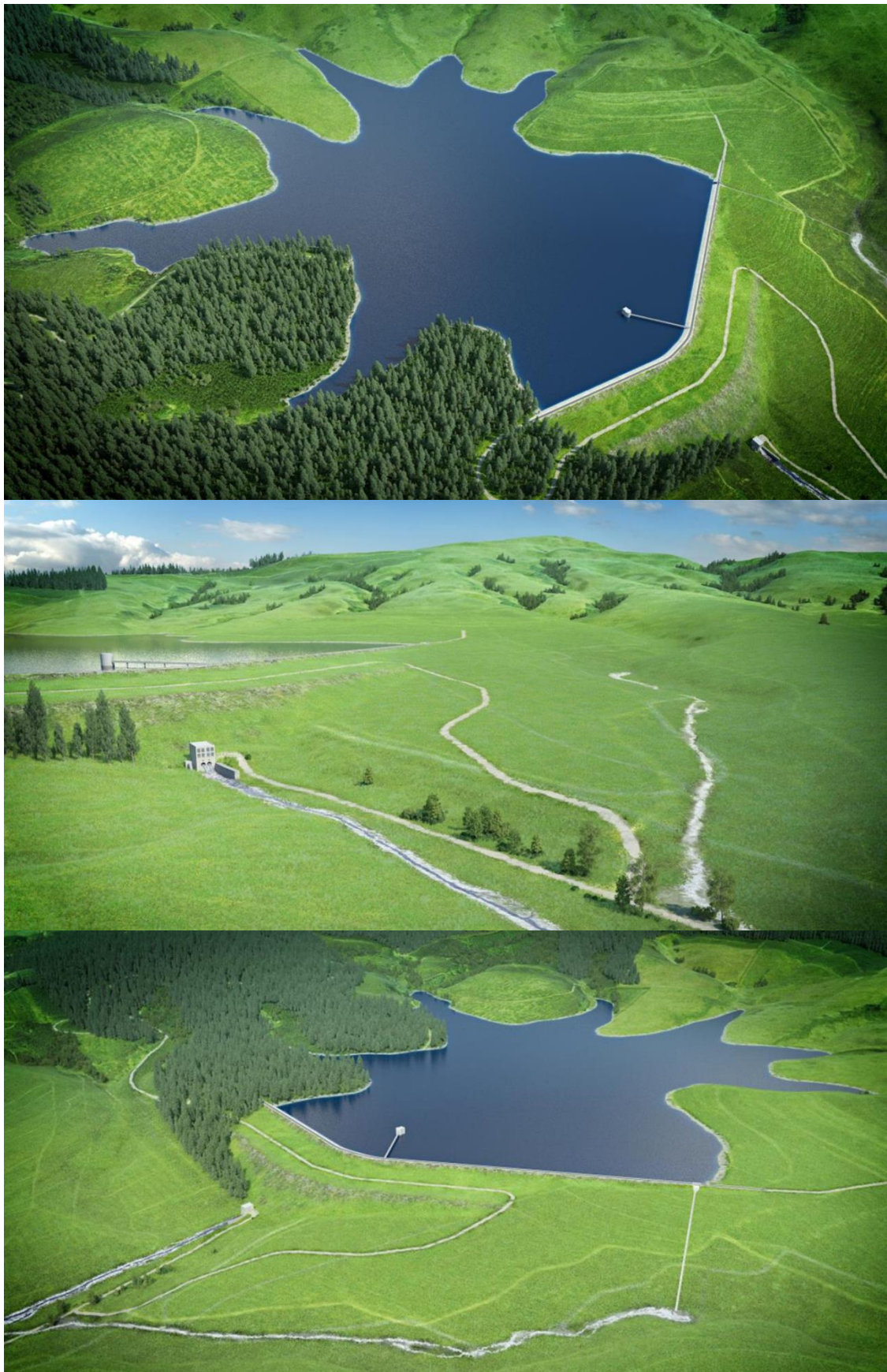
Figure 7.5: Artistic impressions of the alternative vegetation downstream slope for the proposed Langa Dam
